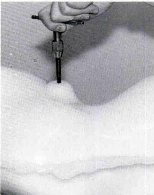
Figure 11. A tap is used to clear the threads and align the holes.
