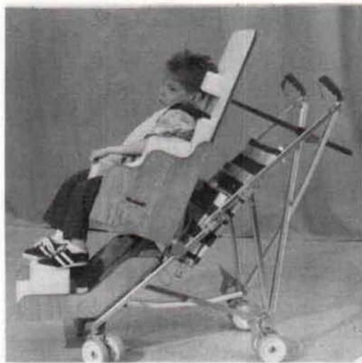
Fig. 4. The MacLaren Buggy Major and patient in orthopedic seat insert in reclined position.
