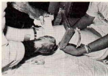
Figure 10 Plastering knee hinges in place.
