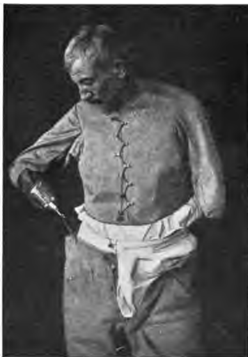
FIG. 172.—A patient with double amputation showing the vest and trousers designed by Spitzzy and a type of artificial arm attachable directly to the clothing. Note the ring hanging down from the slit of the trousers. By pulling this upward with the hook of the artificial arm, the trousers are closed by means of a thin chain with interlocking teeth.
