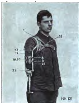
FIG. 136.—Showing adjustment of working arm.
