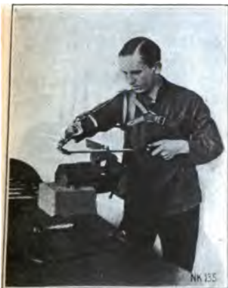
FIG. 140.—Shortened ball connection, with loose file holder.
