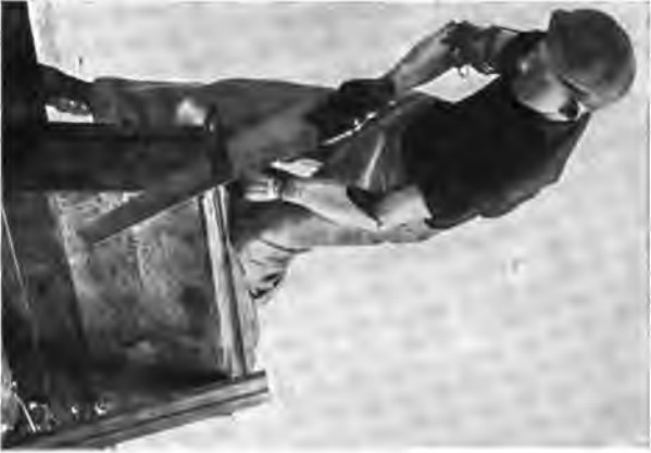
The Carnes artificial arm for the patient shown in Fig. 23.
