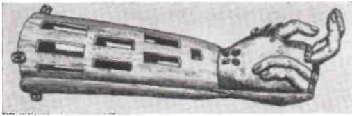
Fig. 3. Alt-Ruppin Hand (circa 1400). The thumb is rigid; the fingers move in pairs and are sprung by the buttons at the base of the palm; the wrist is hinged. From Putti, V., *Chir. d. org. di movimento*, 1924-25.
