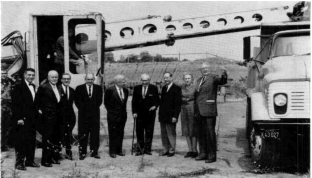
Power shovel scoops up first load of earth at groundbreaking ceremony for UCLA Rehabilitation Center. Left to right: Dr. Ralph Worden, Welton Becket, Dean Sherman Mellinkoff, Vice-Chancellor William G. Young, Associate Dean John Field, Lawrence Frank, Zeb Gullidge, Mary E. Switzer, and Dr. Stafford Warren. UCLA Prosthetics-Orthotics Education will be among the programs conducted at the Center upon its completion.
